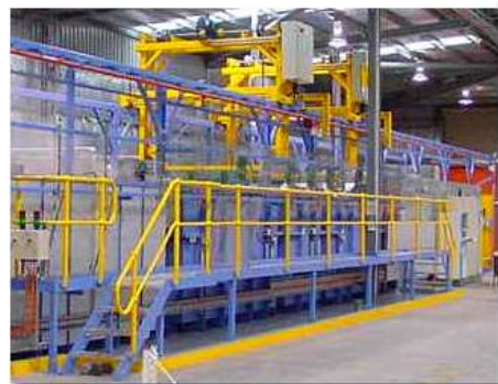
Steelwork and decking installation.
